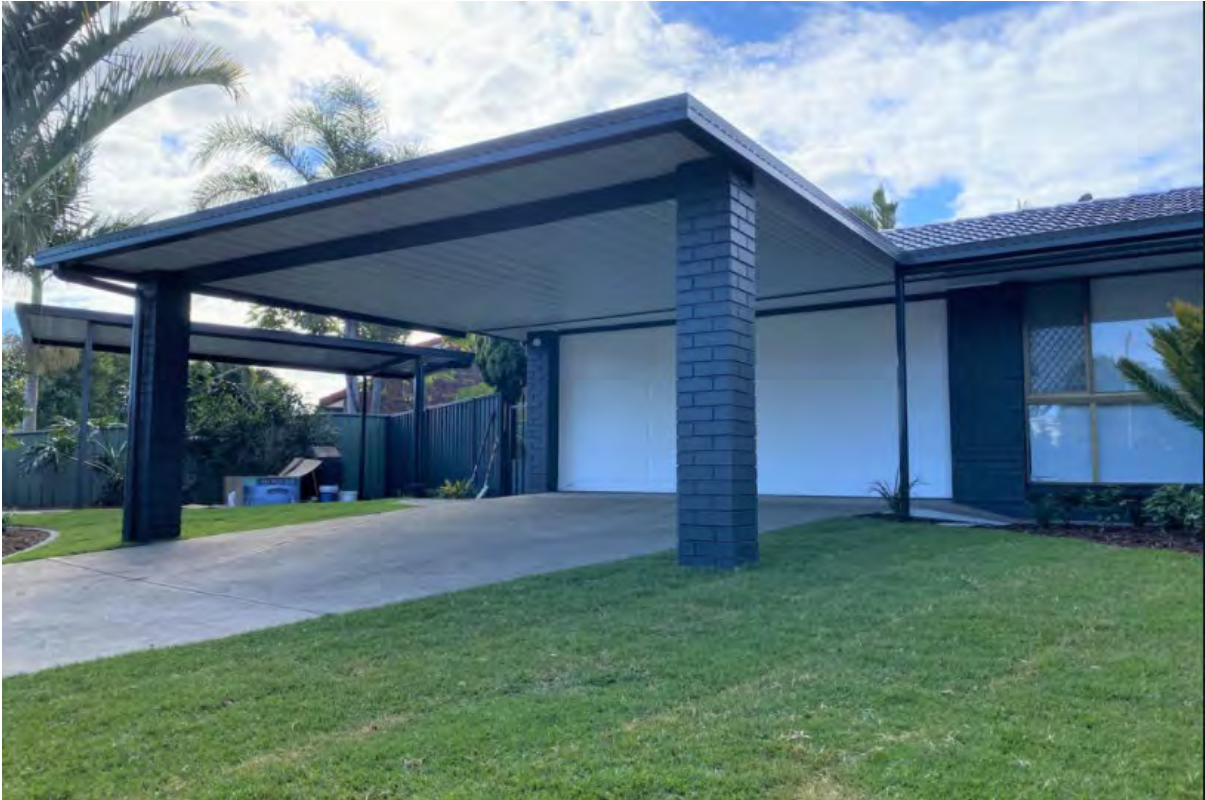
Example 5 – Flat roof carport with brick piers in front of dwelling. Colours match painted walls of house.
