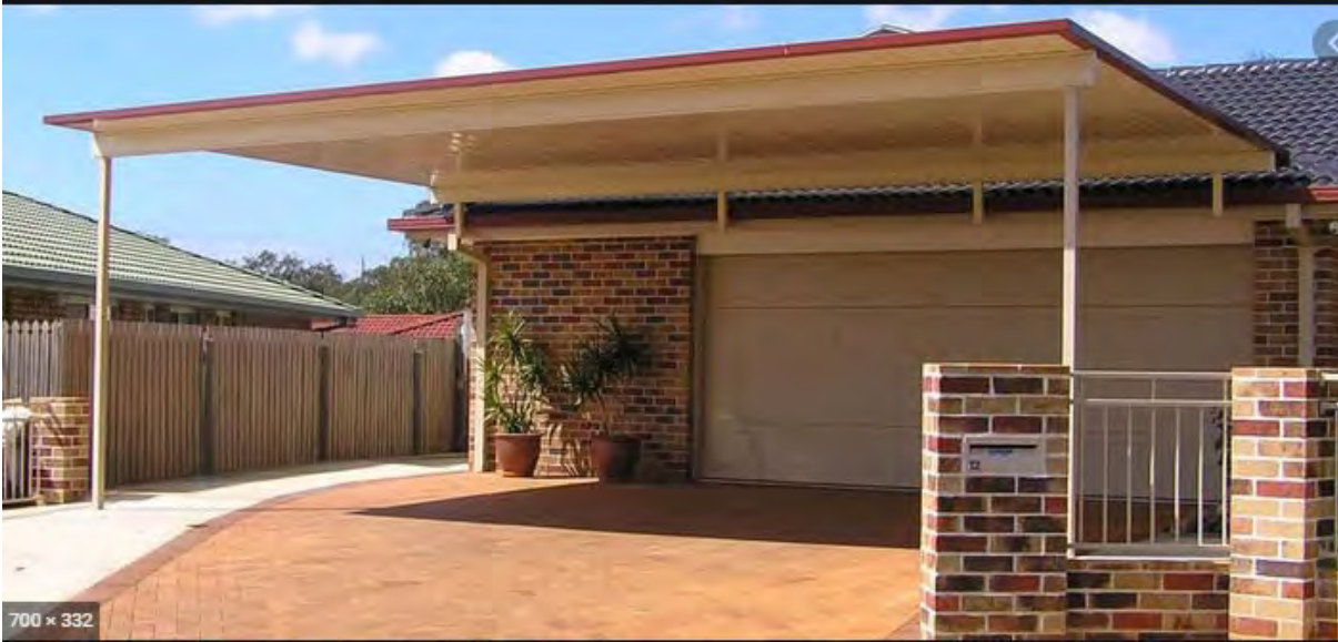
Example 1 – Flat roof carport in front of pitched roof dwelling. Colours match house downpipes/gutters.
