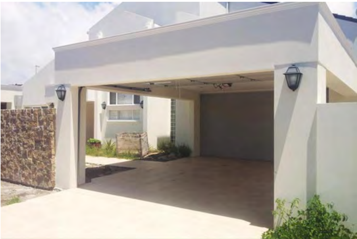
Example 6 and 7 – Flat roof carport with rendered piers in front of dwelling. Colours match rendered house walls.
