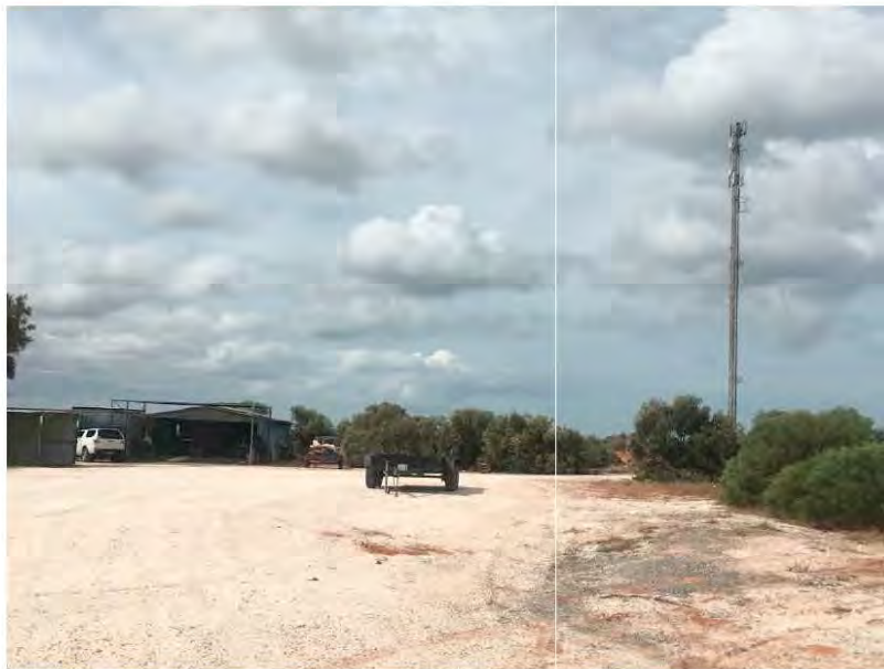
PHOTO 4 - Viewing South from the existing Northwest entry to The Site
