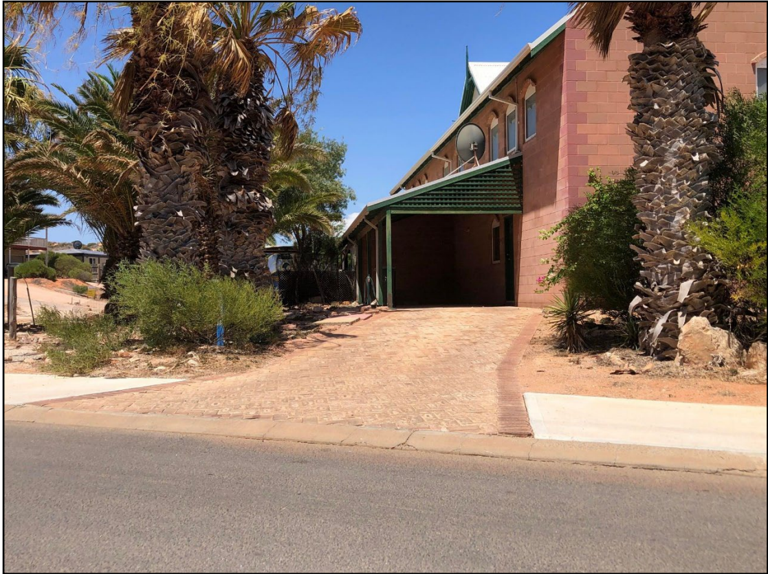
Existing brick paved driveway and carport
