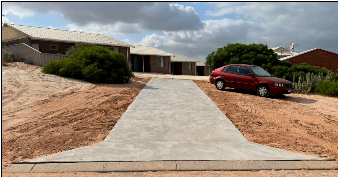
Above: Constructed crossover
