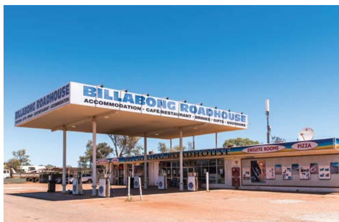
The original and historic Billabong Roadhouse. Credit: Damian Lugowski.
