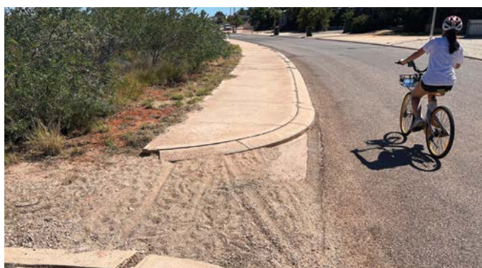
Drainage/spillway channels disrupting path continuity in Exmouth.
