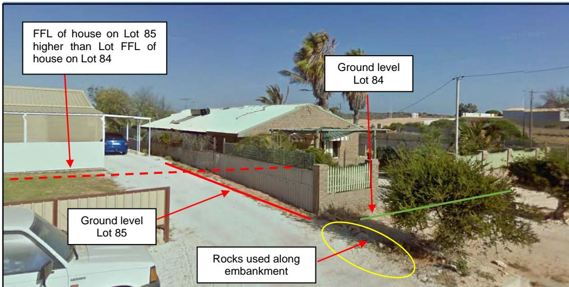
A 0.8 metre high retaining wall is proposed along the southern boundary of Lot 85, to retain the difference in ground levels (with adjacent Lot 84). The retaining wall has no privacy implications as the levels are pre-existing.
