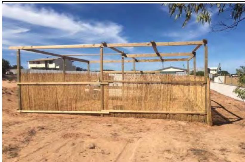
The pergola measures 7.2 metres (width) by 7.2 metres (depth) with a height of 2.96 metres – site plan and elevations below.
