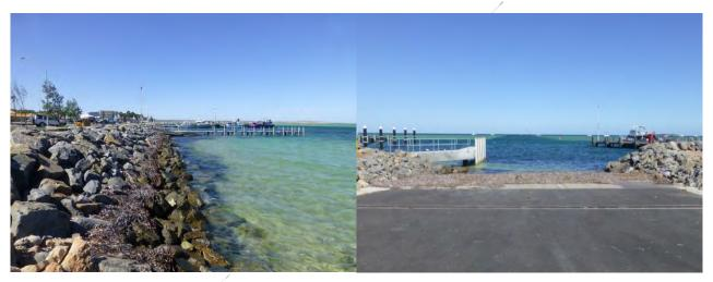
FIGURE 3-8 TYPICAL SECTION OF ROCK ARMOUR REVETMENT ALONG SECTION 3 (LEFT); COMMERCIAL BOAT LAUNCHING RAMP WITH SOME SEAGRASS WRACK ACCUMULATION (RIGHT)
