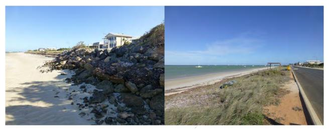
FIGURE 3-4 ROCK SEAWALL WITH VARIABLE ARMOUR SIZING PROTECTING KNIGHT TERRACE TURNAROUND (LEFT); TYPICAL BEACH PROFILE IN SECTION 1 (RIGHT)
