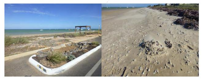
FIGURE 3-5 ROAD TO BEACH DRAINAGE INTERFACE ON KNIGHT TERRACE (LEFT); BEACH FACE SHOWING EVIDENCE OF AEOLIAN SEDIMENT TRANSPORT
