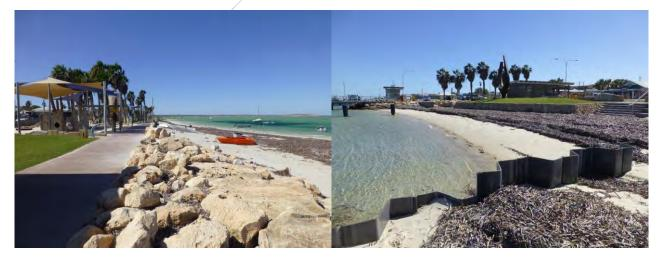
FIGURE 3-7 WIDE BEACH AND IMPROVED ARMOUR STRUCTURE IMMEDIATELY ADJACENT TO FRP GROYNE (LEFT); LANDWARD END OF FRP GROYNE AND SMALL BEACH SECTION UP TO (RIGHT)
