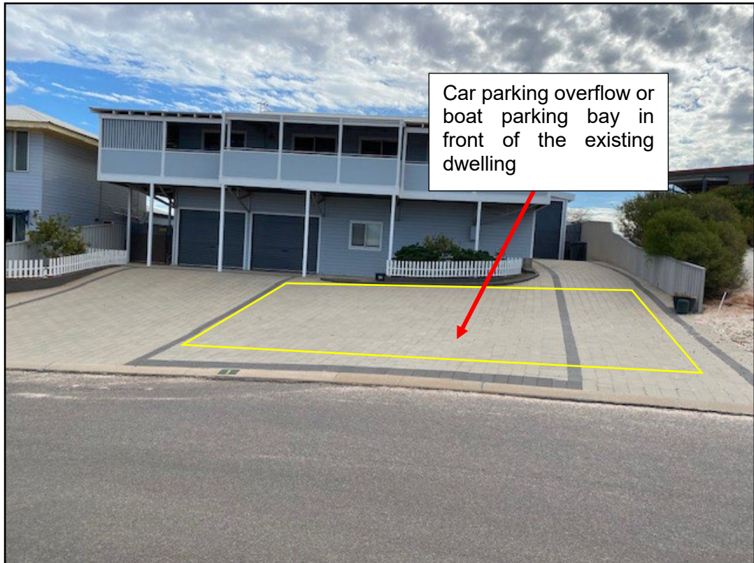
Above: Photo showing over flow parking or boat parking bay
