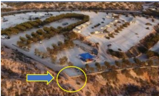
Figure 4: Boundary Fence Encroachment
