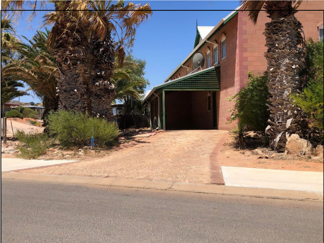
Existing brick paved driveway and carport
