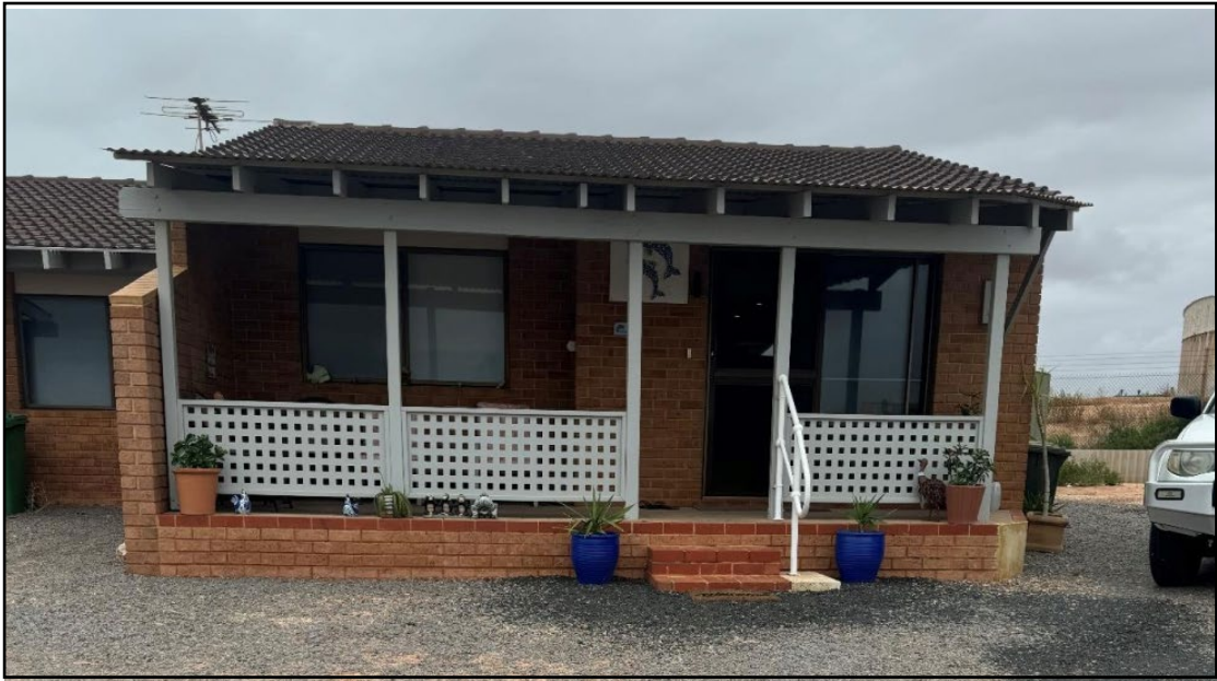
Above: Right hand side (eastern) unit
