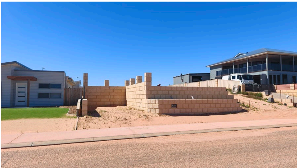
Above and below: View of retaining walls on Lot 15 and existing house with outbuilding on Lot 16
