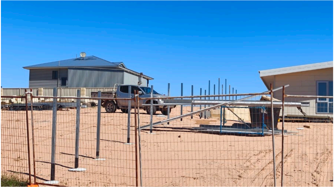
Above: View of Lot 15 and 16 from the rear. Department of Housing premises on Lot 4 is shown on the right.
