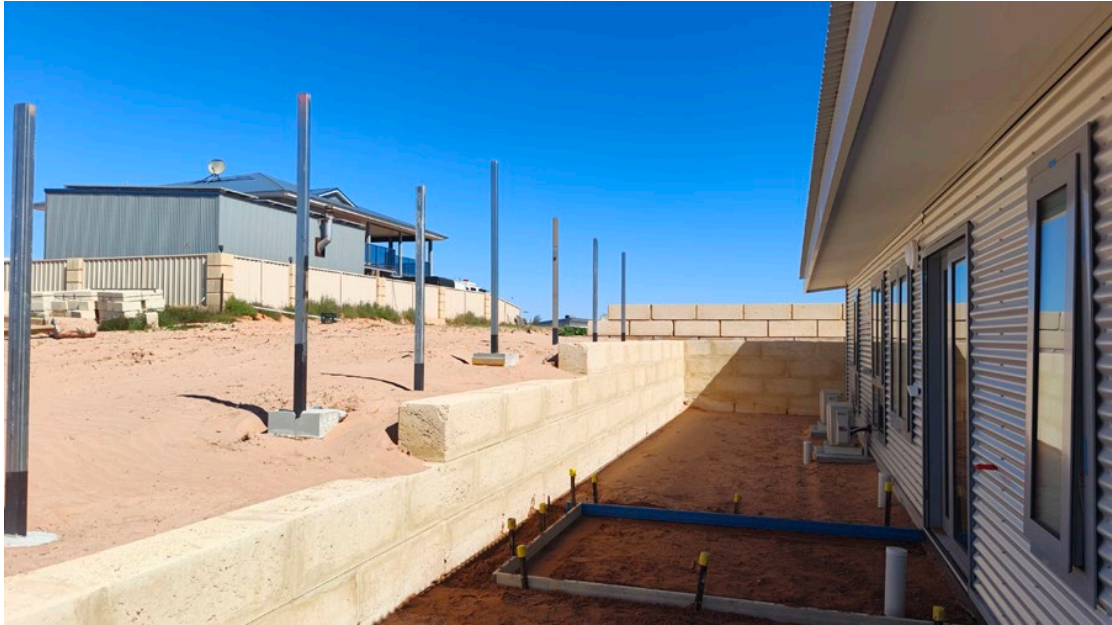
Above: View of existing outbuilding from Lot 4.
