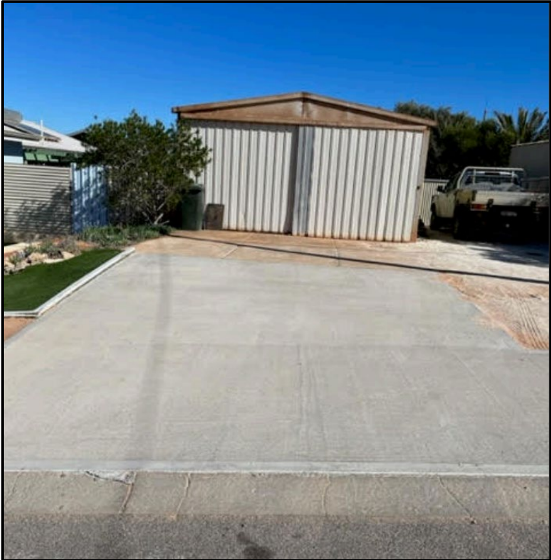
Above: Constructed crossover
