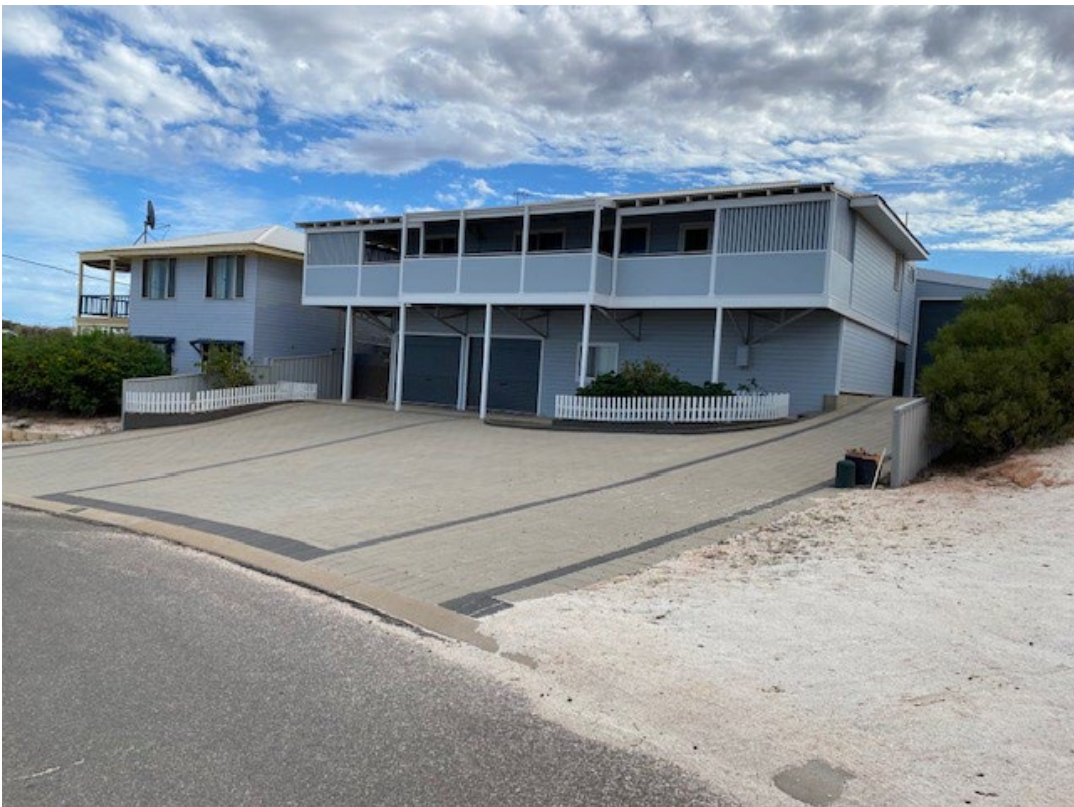
Above: Photograph of existing dwelling as viewed from Leeds Court
