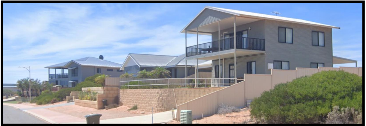
Above: Existing retaining walls at 6 and 8 Terry Deschamps Way
