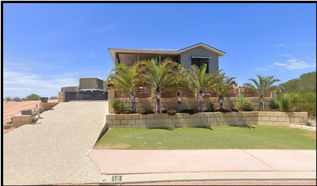
Above: Existing development on Lot 15.
