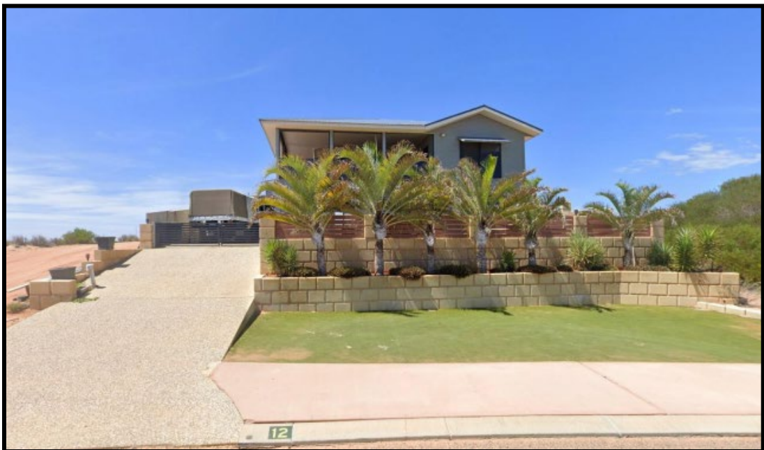
Above: Existing development on Lot 15.
