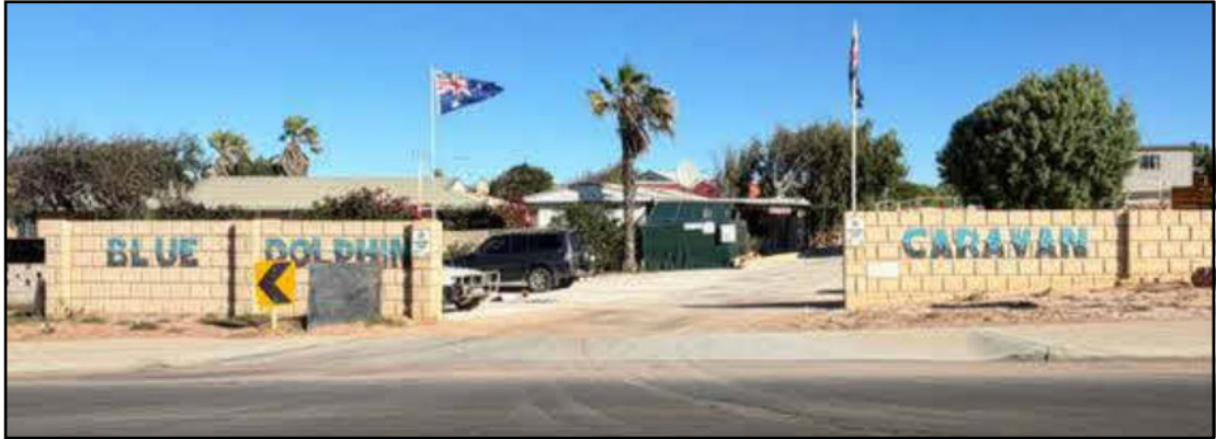
Above: Limestone entry walls in Denham Road, road reserve
