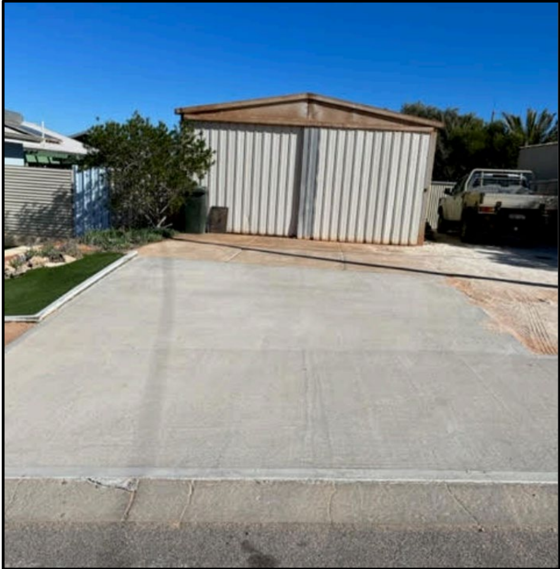
Above: Constructed crossover
