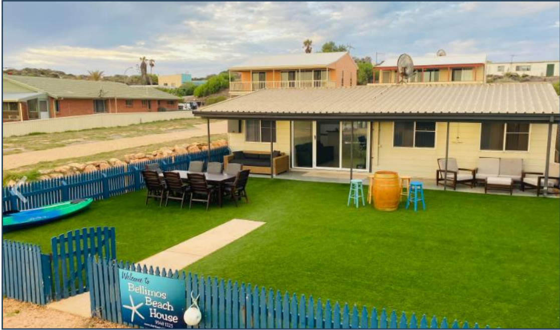
Above: Photograph of existing dwelling at 19a Knight Terrace Source: Ray White website
