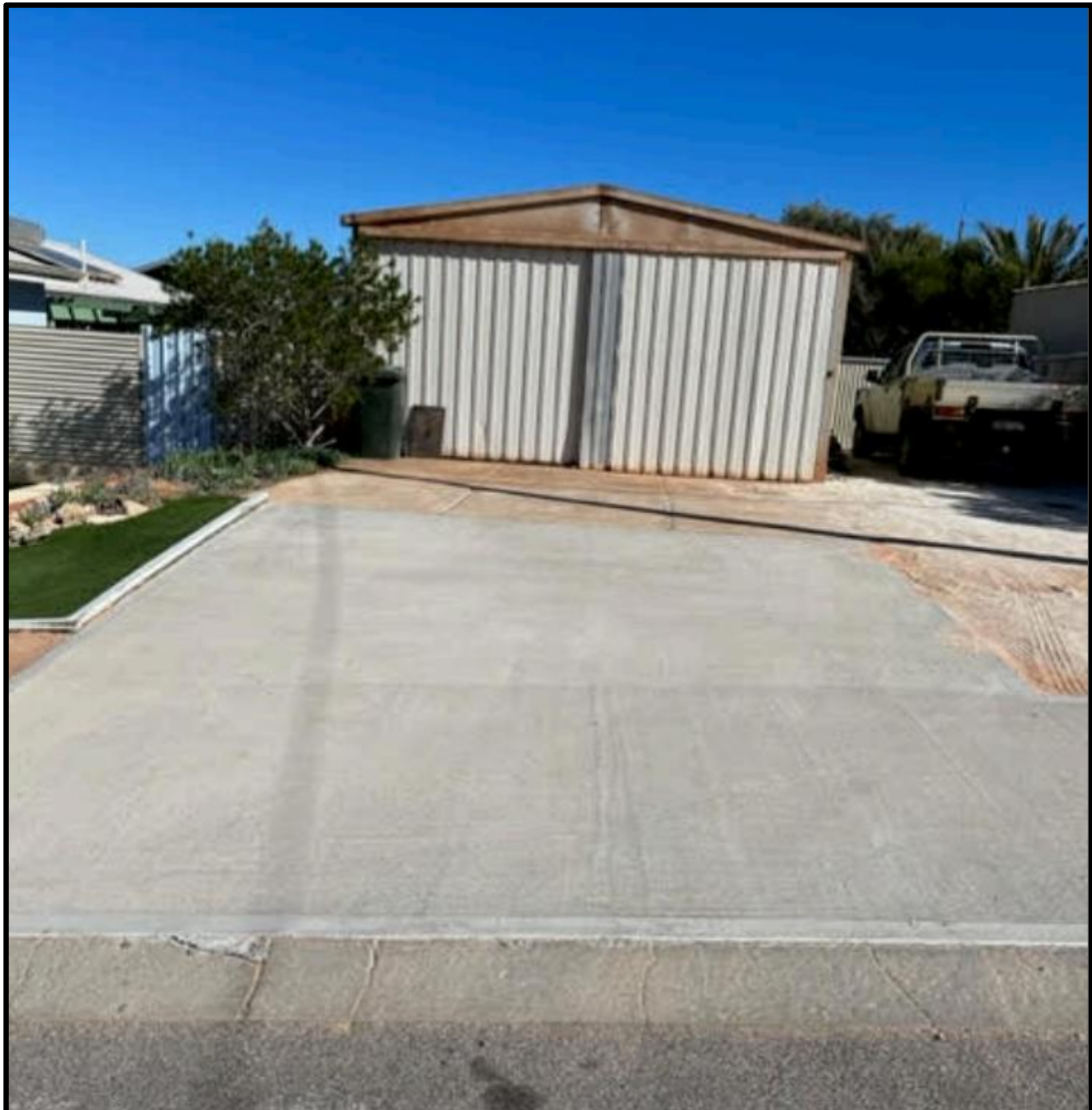
Above: Constructed crossover
