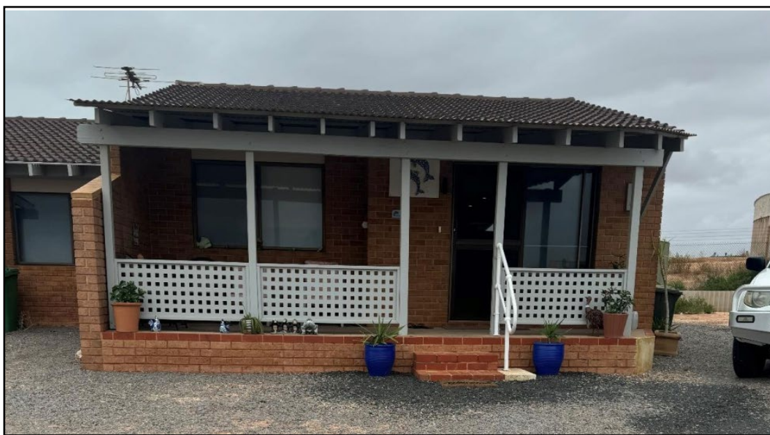
Above: Right hand side (eastern) unit
