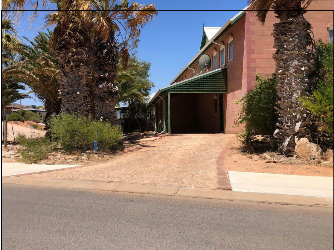
Existing brick paved driveway and carport
