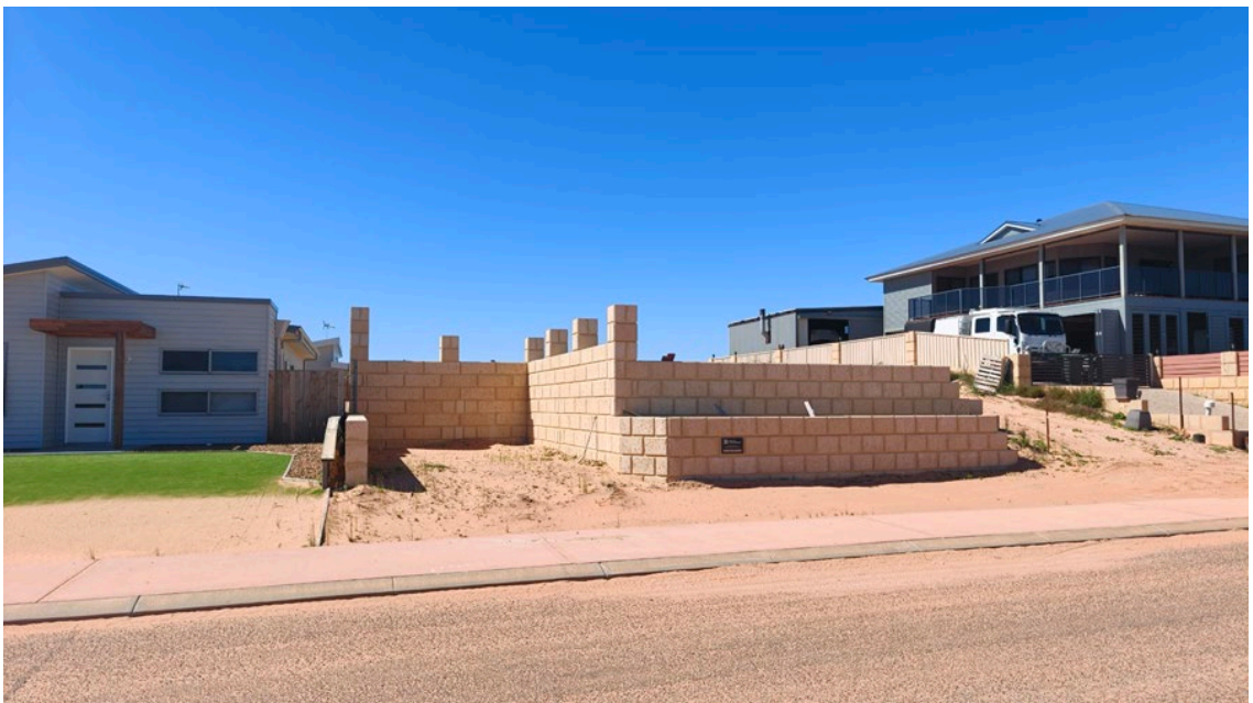
Above and below: View of retaining walls on Lot 15 and existing house with outbuilding on Lot 16
