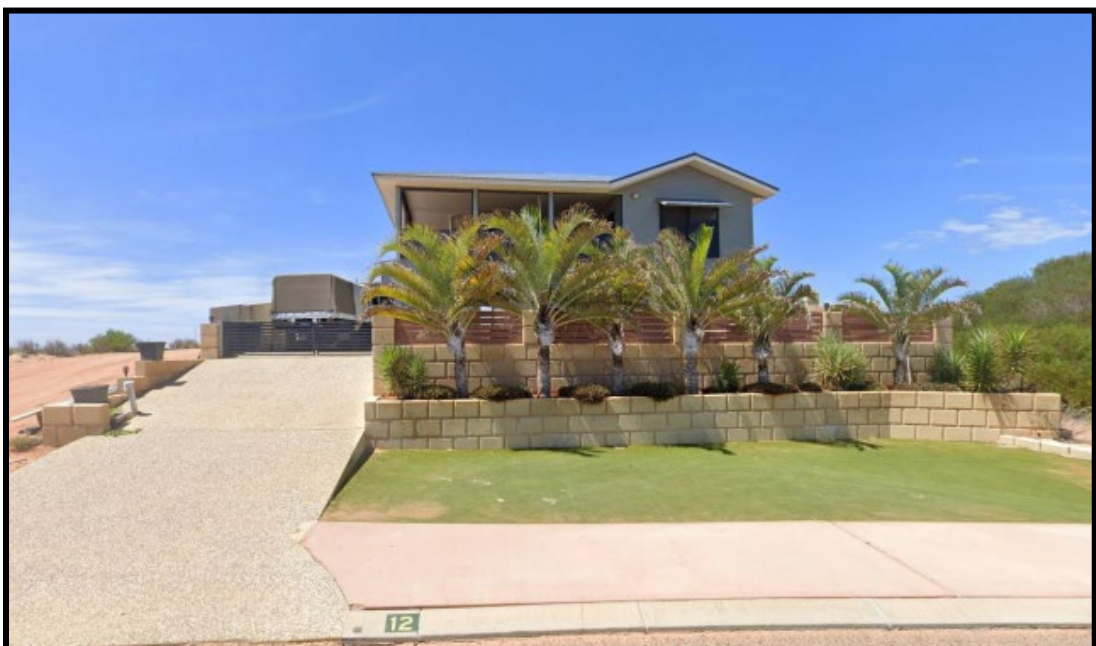
Above: Existing development on Lot 15.
