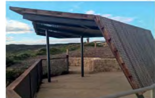
Timber batted structure to provide dappled shade and a welcoming area
