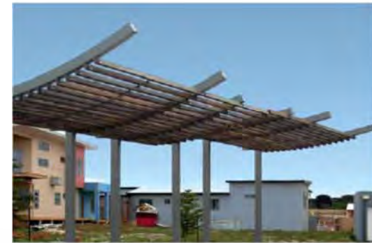
Timber battens in wave form to provide dappled shade and allow for drainage
