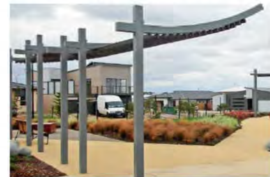
Timber battens to provide dappled shade and allow for drainage
