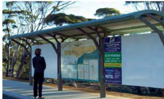
Dundas Information Shelter
