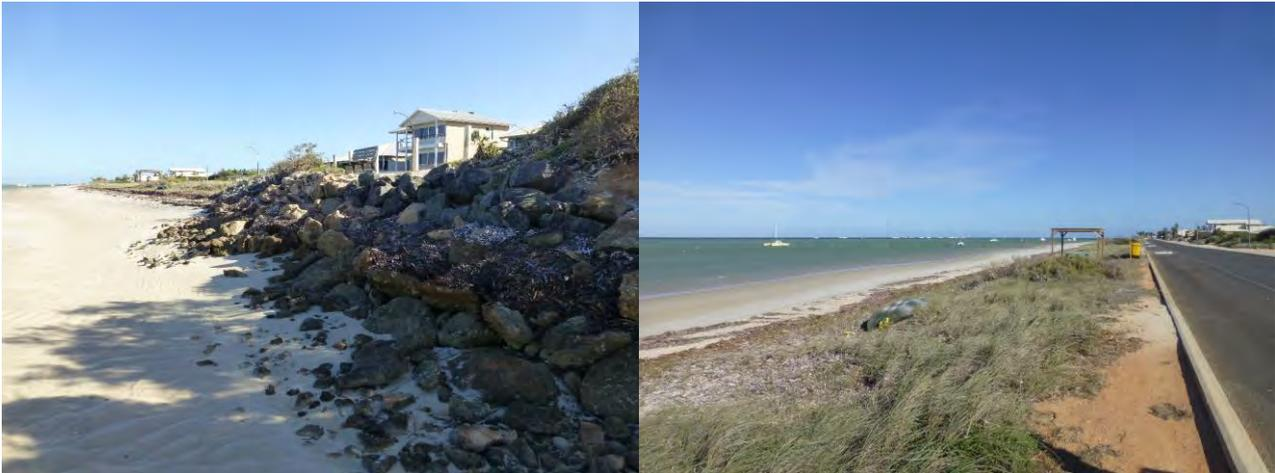
**FIGURE 3-4 ROCK SEAWALL WITH VARIABLE ARMOUR SIZING PROTECTING KNIGHT TERRACE TURNAROUND (LEFT); TYPICAL BEACH PROFILE IN SECTION 1 (RIGHT)**
