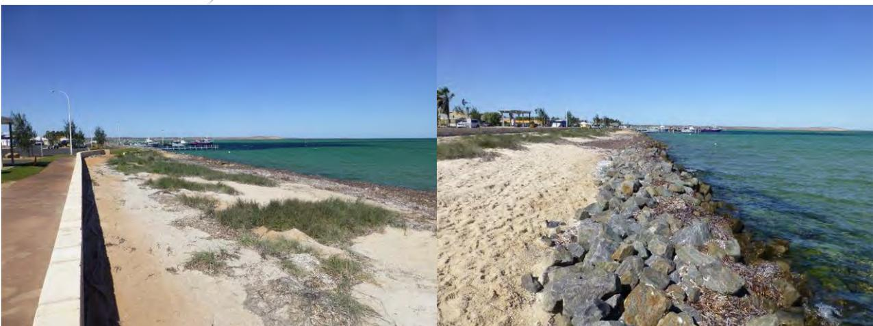
**FIGURE 3-9 NORTHERN HALF OF SECTION WITH LOWER CRESTED SEAWALL AND SPARSELY VEGETATED BEACH**
