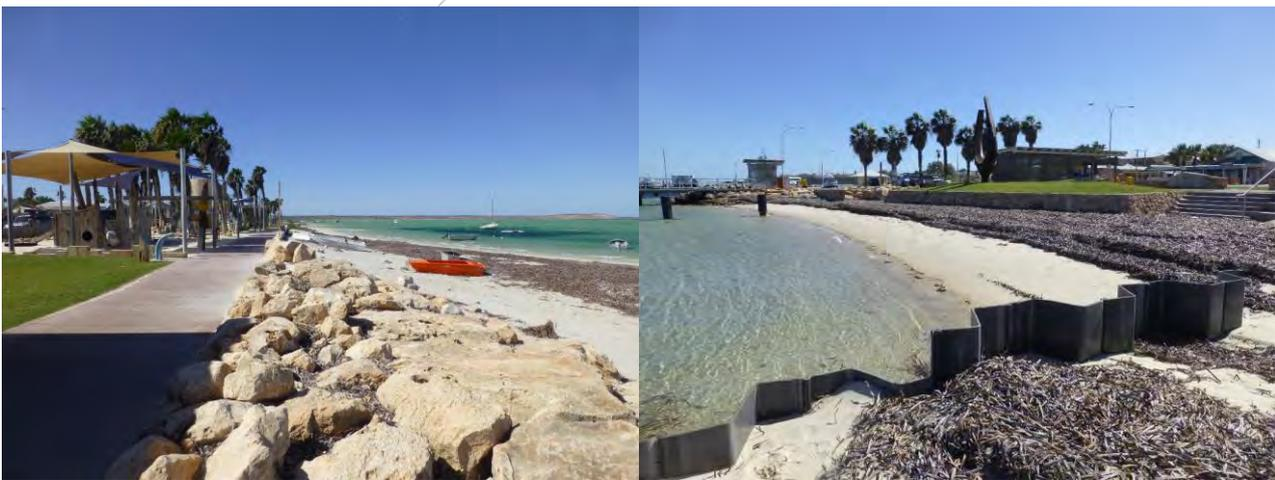
**FIGURE 3-7 WIDE BEACH AND IMPROVED ARMOUR STRUCTURE IMMEDIATELY ADJACENT TO FRP GROUYNE (LEFT); LANDWARD END OF FRP GROUYNE AND SMALL BEACH SECTION UP TO (RIGHT)**
