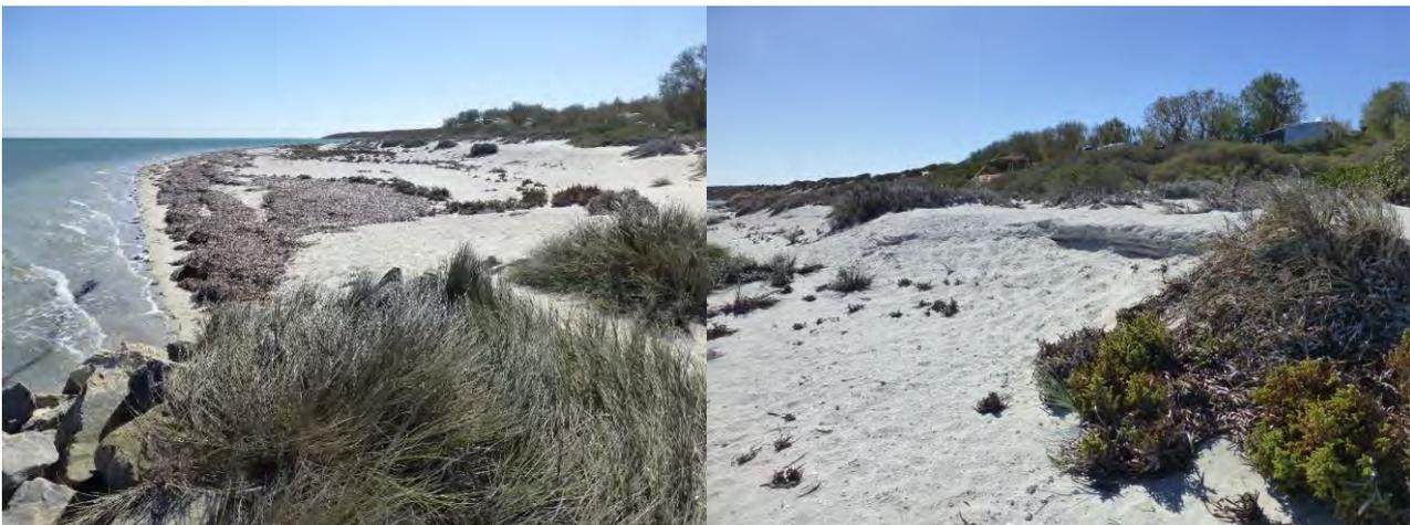
**FIGURE 3-10 SOUTHERN EXTENT OF SECTION 4 VIEWED FROM THE REVETMENT TIE-IN. RECENT RENOURISHMENT AND PRE-NOURISHMENT SHORELINE VISIBLE (LEFT); SECTION OF EXPOSED SCARP REPRESENTATIVE OF THE 1956 SHORELINE LOCATION (RIGHT)**
