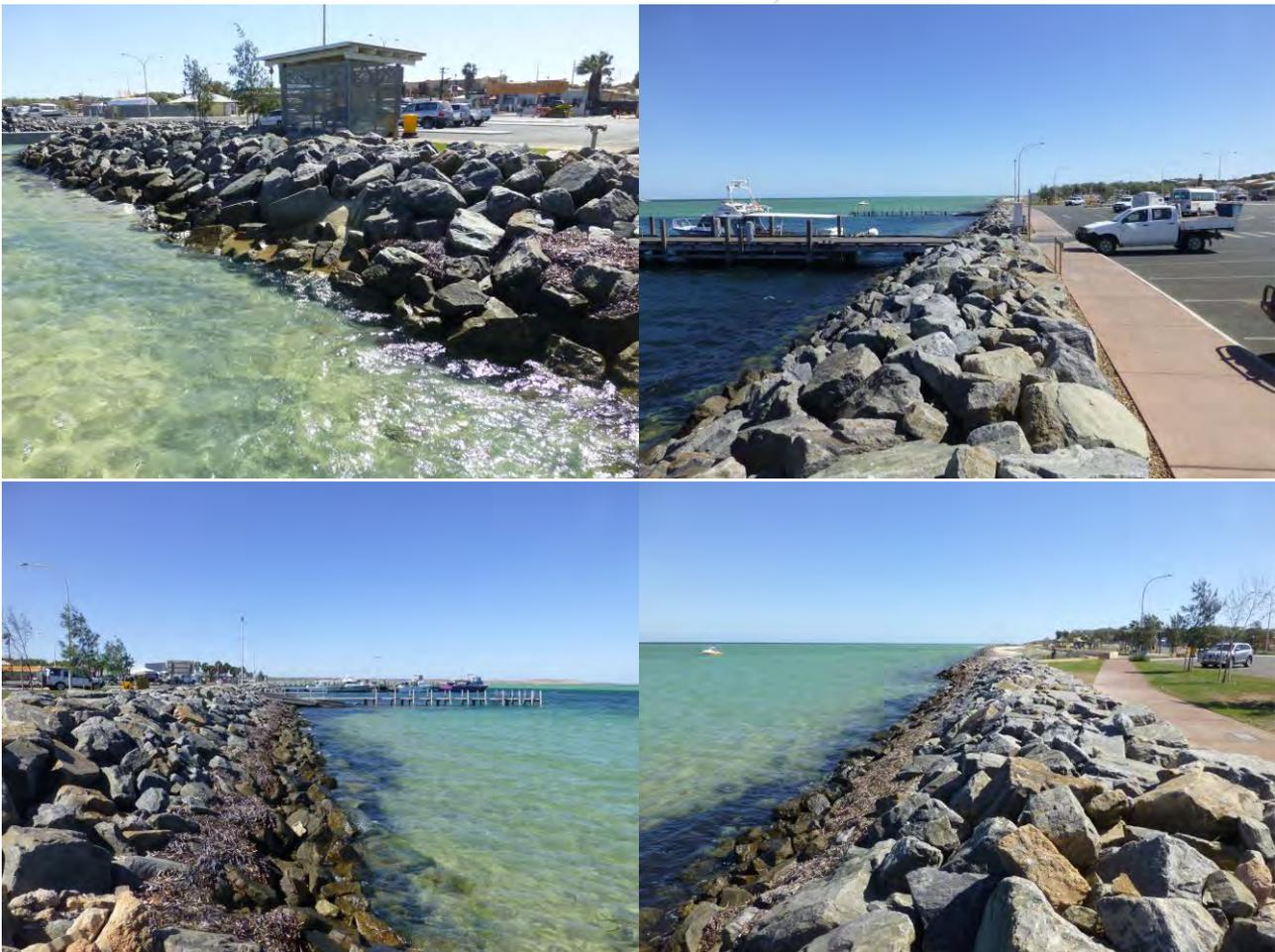
FIGURE 5-2 ENGINEERED SEAWALL ALONG FORESHORE
