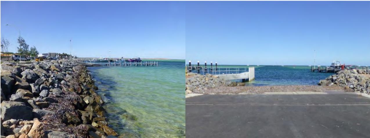
**FIGURE 3-8 TYPICAL SECTION OF ROCK ARMOUR REVETMENT ALONG SECTION 3 (LEFT); COMMERCIAL BOAT LAUNCHING RAMP WITH SOME SEAGRASS WRACK ACCUMULATION (RIGHT)**
